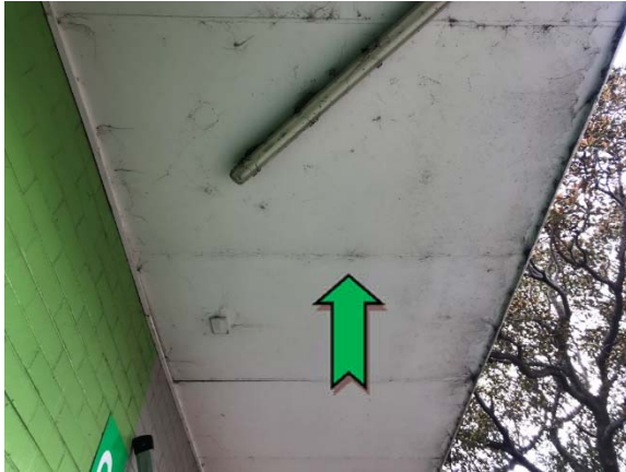
Photo 1. Exterior, south-east elevation, awning – non asbestos-containing fibre cement sheeting.
